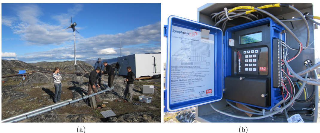
Figure 2.3: Work on the old met. mast at Sarfannguaq. (a) Cabling and anemometers mounting - (b) Configuring the new data-logger with i-Pack
